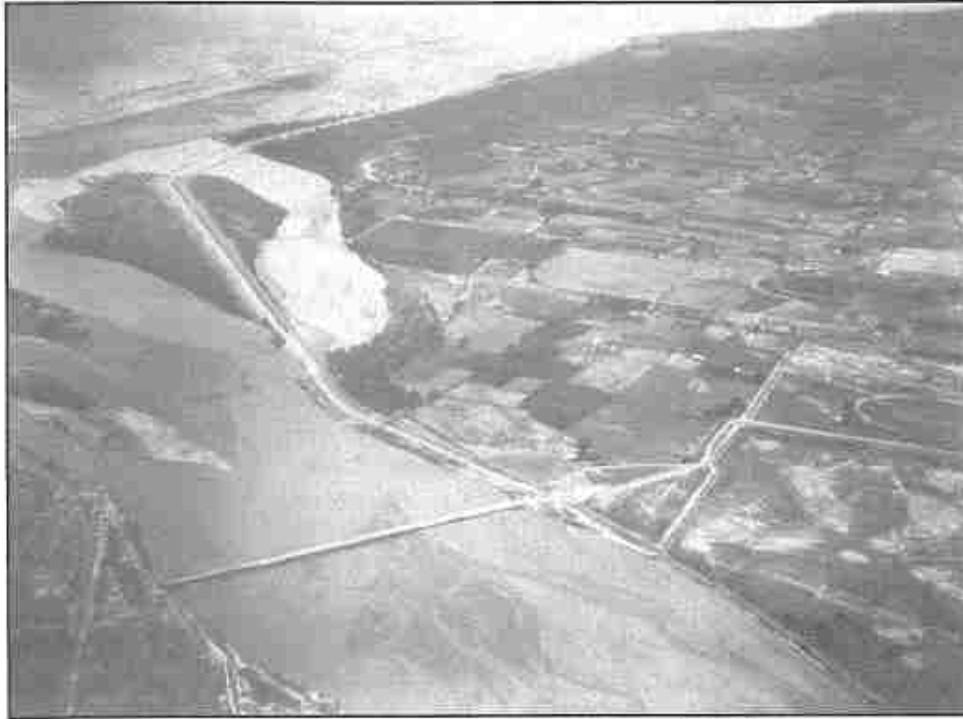
Figure 21: Central Avenue Bridge on May 26, 1930 (from Daves, 1994).
